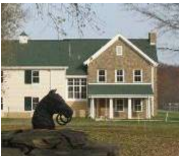
The Inn nears completion.
